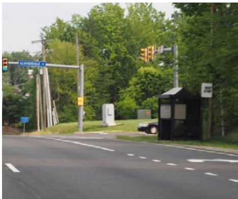
Existing near-side bus stop without sidewalk access is difficult to access and conflicts with right turns.
