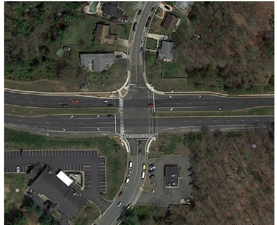
Curb extension and Continental (zebra) striped crosswalks at Dale Boulevard and Forestdale Avenue.
