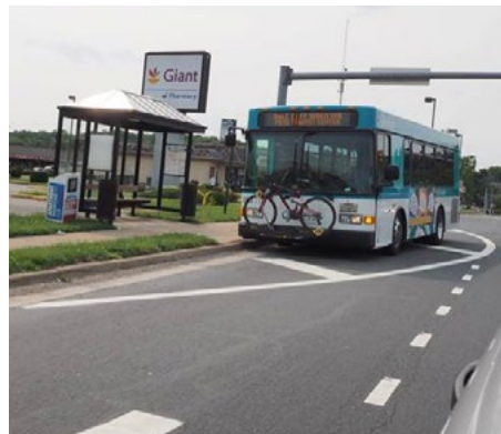
Existing far-side bus stop with sidewalk access is easier to access and does not conflict with right turns or through traffic.
