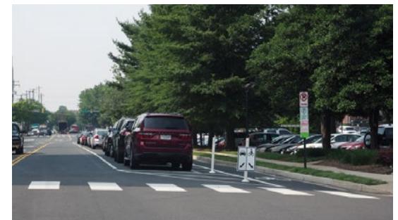
Protected or separated bike lanes ( aka “cycle tracks”) with raised curb and stormwater collection buffer (upper images) and striped buffer with bollards (lower images).
