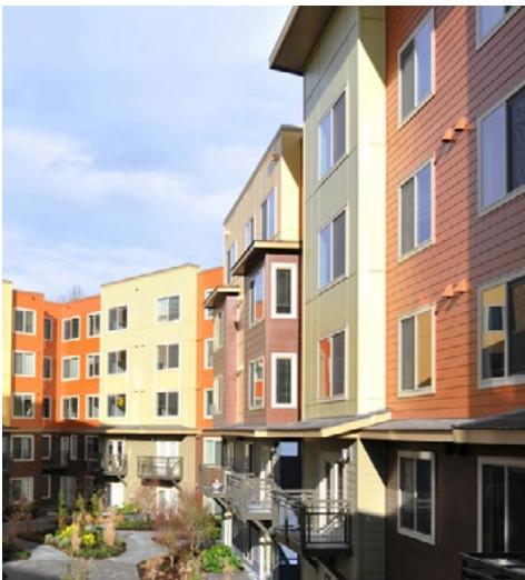
Multi-level senior care residence.
