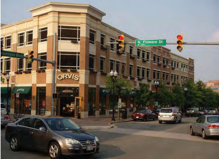
Ground level retail use wrap and compatible façade on upper stories of parking structure
