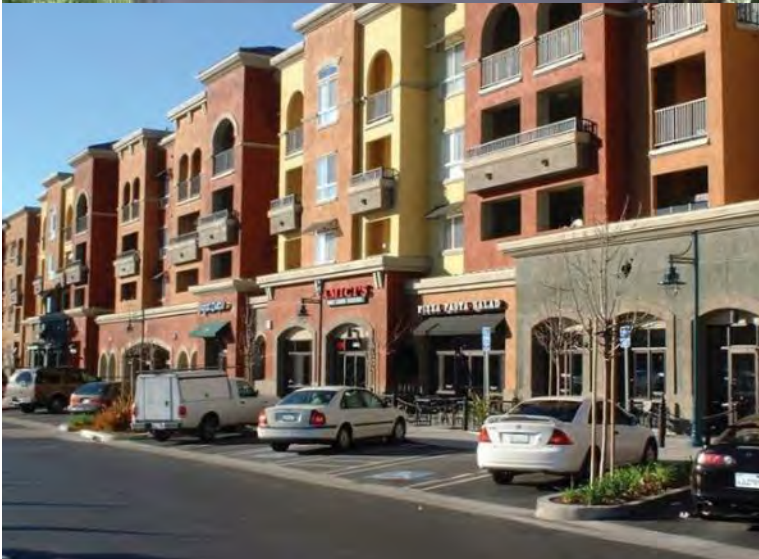
On-street diagonal parking
