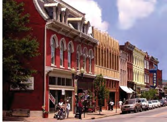
Vertical articulation of buildings
