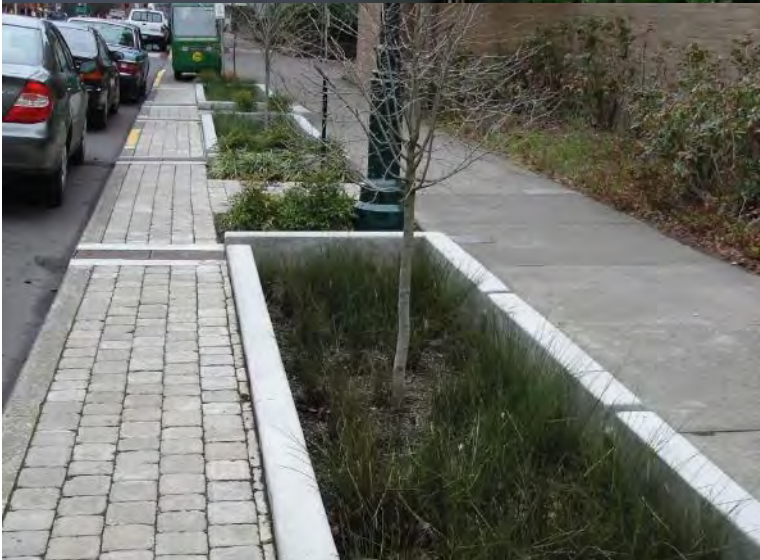
Low impact development (LID) curbside planting strips creating a buffer between the roadway and the sidewalk
