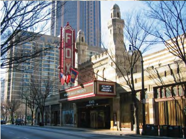
Primary building entry oriented towards street
