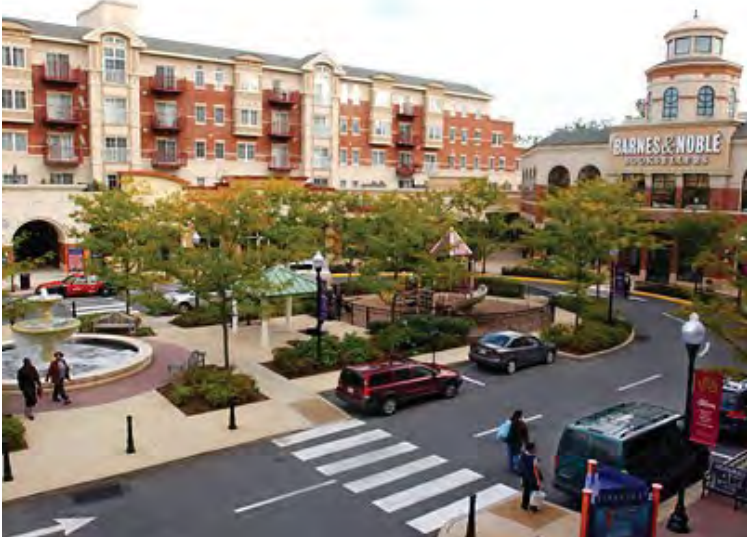
Creation of new perpendicular street/access drive to achieve adequate building orientation objectives
