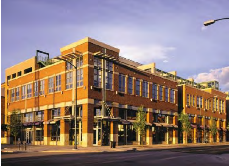
Garage façades create visually interesting façades compatible in character and quality with adjoining buildings, while concealing the impact of parked cars
