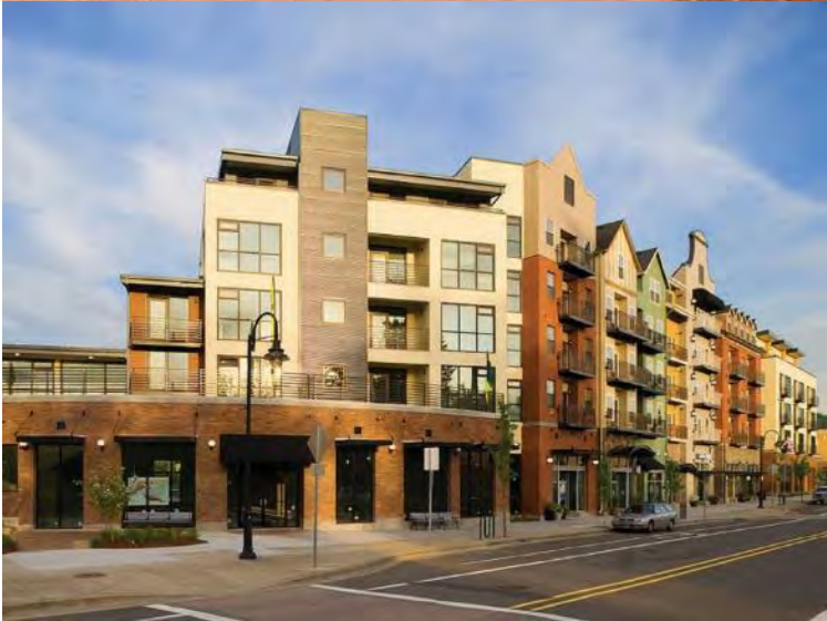
Vertical articulation of buildings
