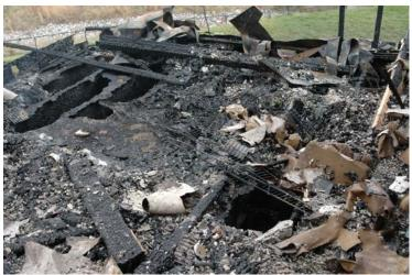
Collapse and hole burn through of second floor bedroom in Quadrant Bravo
