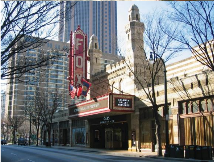
Primary building entry oriented towards street
