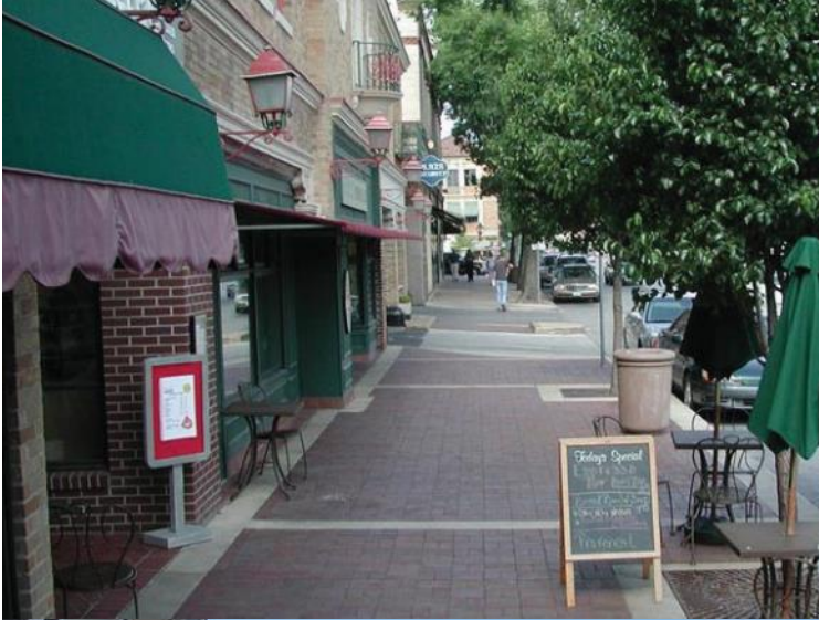
Driveway across sidewalk identified by material change
