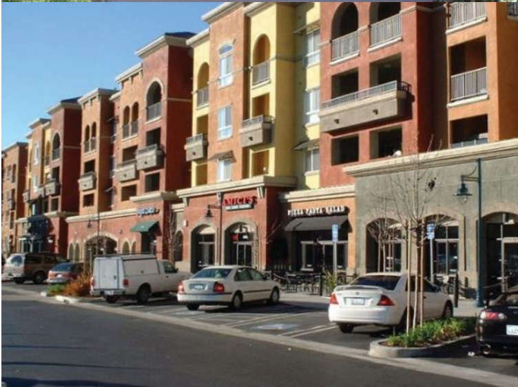
On-street diagonal parking
