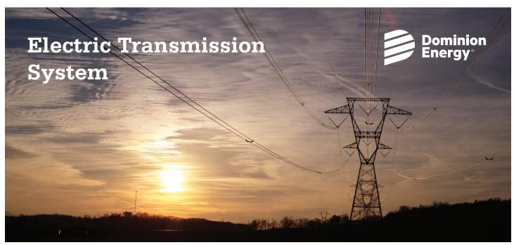
500 kilovolt lattice structure with 230 kilovolt underbuild
