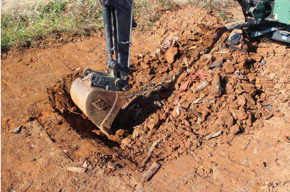
Figure 24. Photograph showing Anomaly F9 excavation in progress showing vast amounts of modern trash within subsurface deposit, facing northwest.
