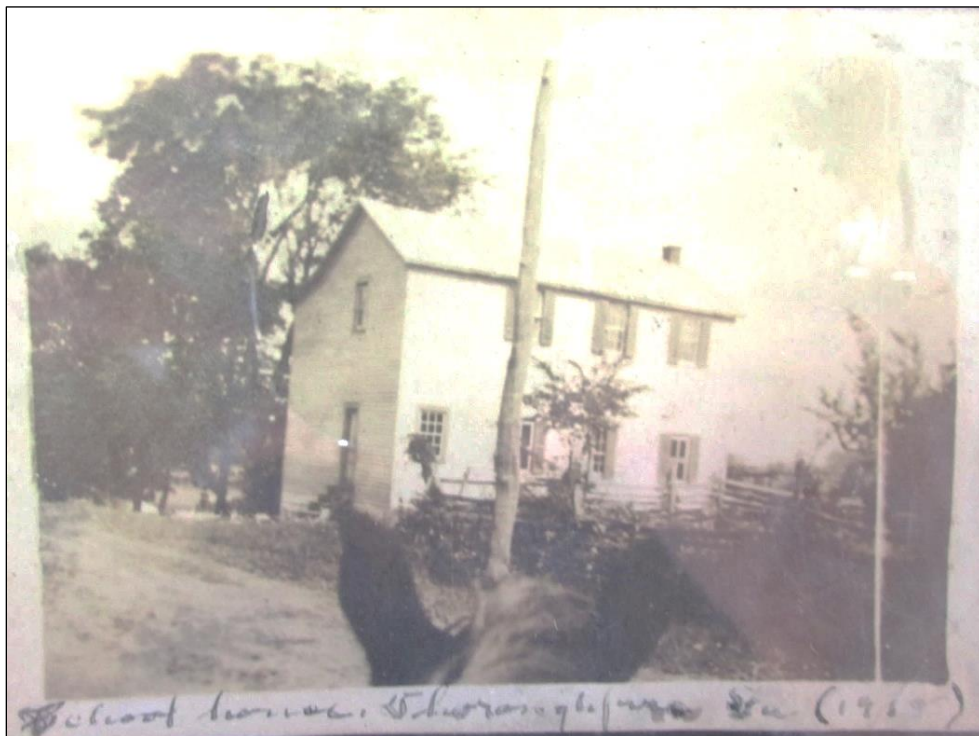
Figure 4: 1918 Photograph of North Fork School, Thoroughfare, Virginia, Courtesy of Donald Christian.
