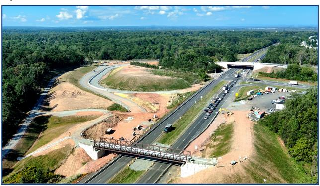
**Fuller Road/Fuller Heights Road Improvements** – This project included improvements to Fuller Road, the access road to the Quantico Marine Corps Base, a new left-turn lane along Joplin Road onto northbound Route 1, conversion of an existing left-turn lane to a thru lane, and the realigning of Fuller Heights Road.
