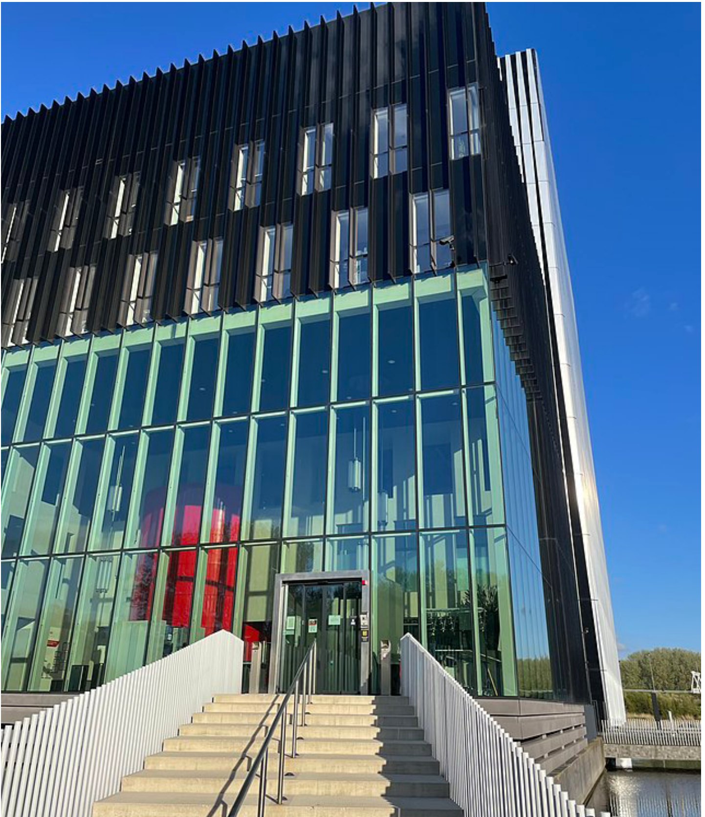
Equinix Data Center, Amsterdam, Netherlands.
