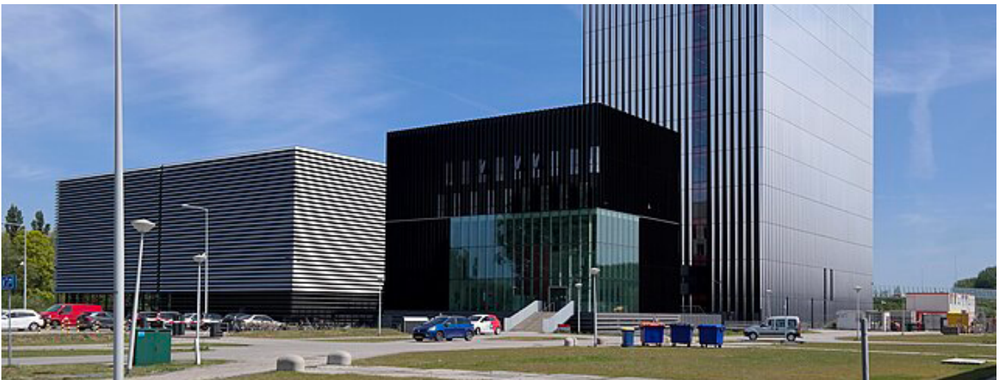
Equinix Data Center, Amsterdam.
