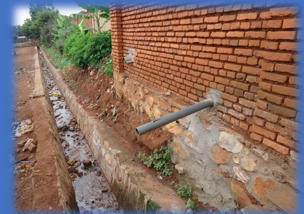
Illegal sewer connection to stormwater drainage | Flickr
