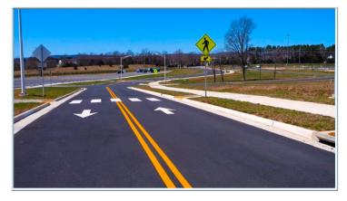
**Long Park Intersection Improvement** – This project involved constructing an additional right-turn lane from Long Park onto Route 15, adjusting the traffic signal, and building a paved parking lot and shared-use path within the park.
