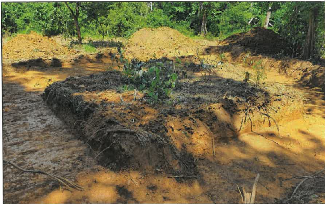
Figure 5-148: Overall view of trench excavations facing northeast.
