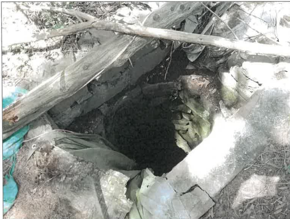
Figure 5-40: Well feature associated with Stone Foundation 1 at site 44PW1590, facing northeast.
