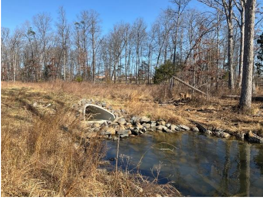
G-1, Culvert outside Study Area
