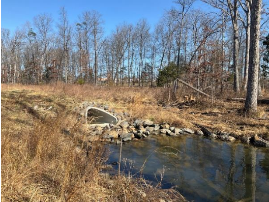
G-1, Culvert outside Study Area
