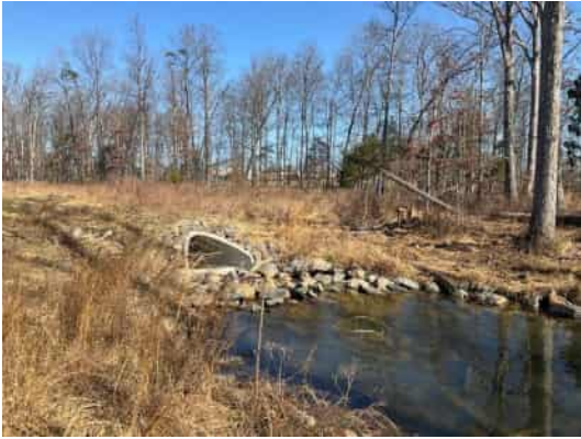
G-1, Culvert outside Study Area
