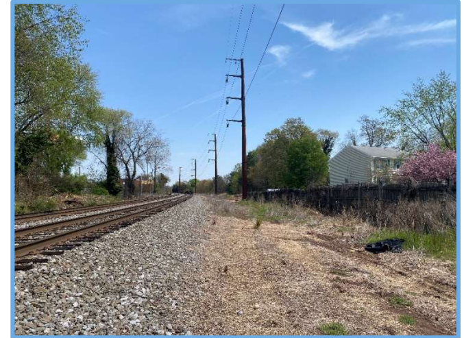
Figure 12: Constrained Area East of Fairview Avenue
