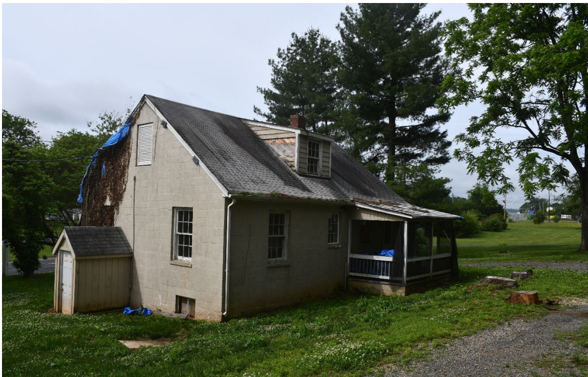
Figure 6: Hazel House, 16210 Lee Highway, Looking Southwest, May 2026
