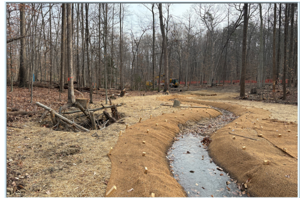
Occoquan River - Chinn Park stream restoration
