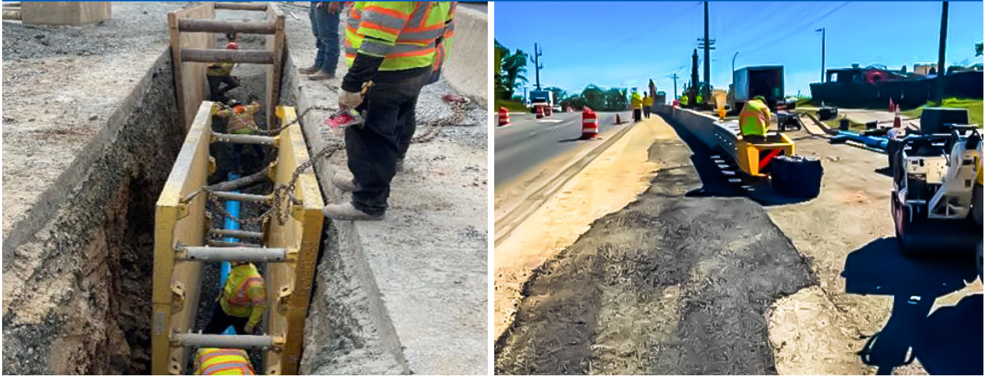
BEFORE & AFTER – Balls Ford Road Sanitary Sewer Project
