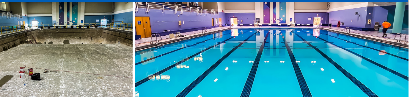
BEFORE & AFTER – Chinn Aquatic Center Pool Whitecoat, Building & Facilities Capital Program
