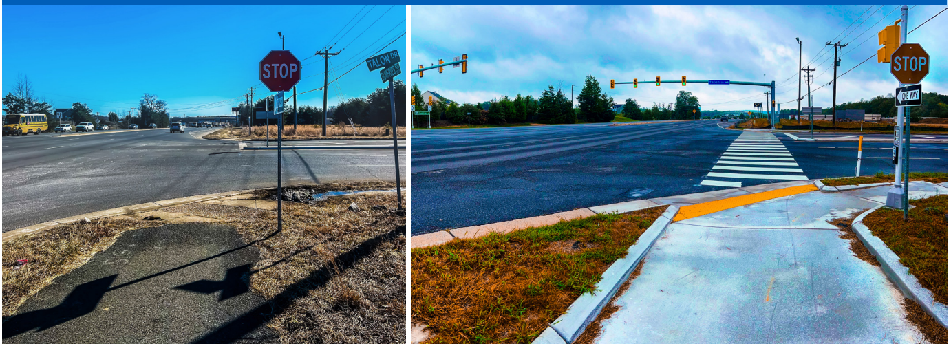
BEFORE & AFTER – Talon Drive – Route 234 Signal Project
