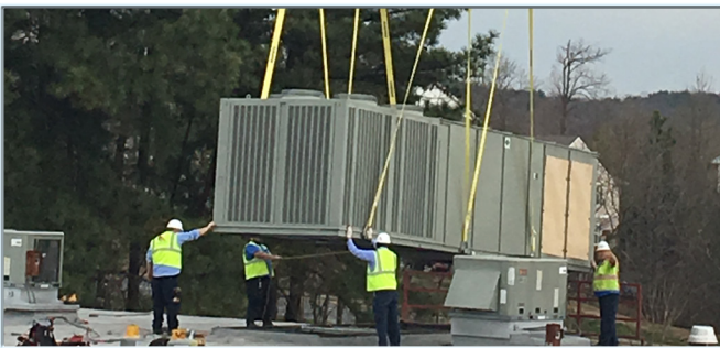
Ferlazzol HVAC Rooftop Unit Replacement
