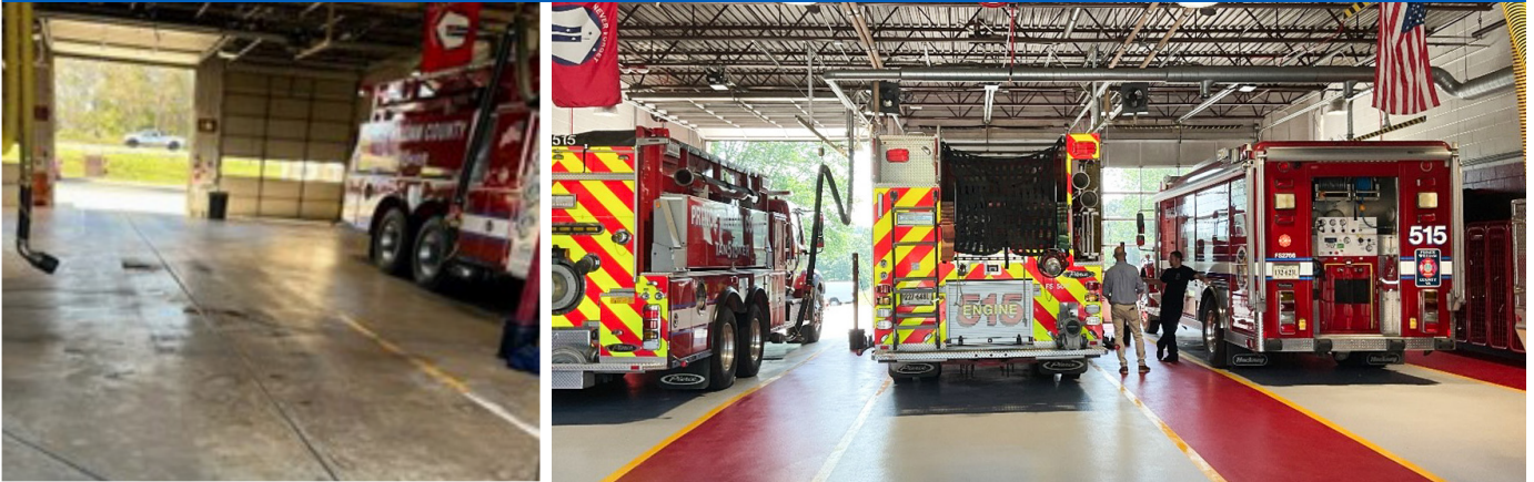
BEFORE & AFTER – Fire Station 15, Fire & Rescue System Station Renovation & Rebuilding Program
