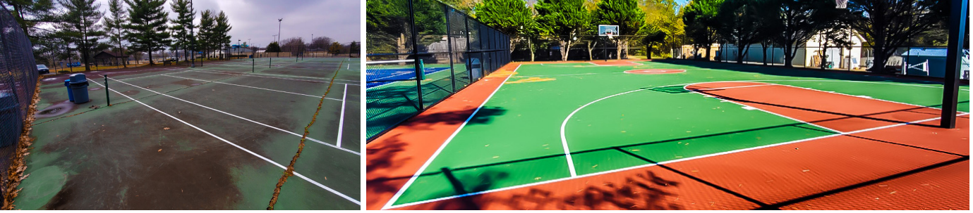
BEFORE & AFTER – SplashDown Waterpark Courts, ARPA
