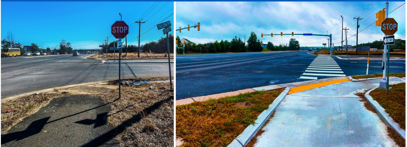
BEFORE & AFTER – Talon Drive – Route 234 Signal Project
