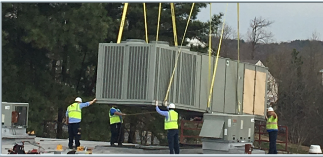
Ferlazzol HVAC Rooftop Unit Replacement
