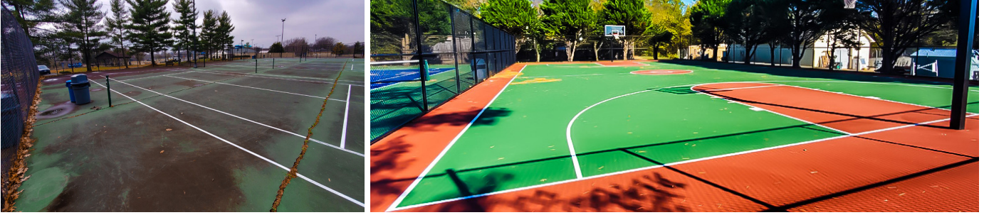
BEFORE & AFTER – SplashDown Waterpark Courts, ARPA
