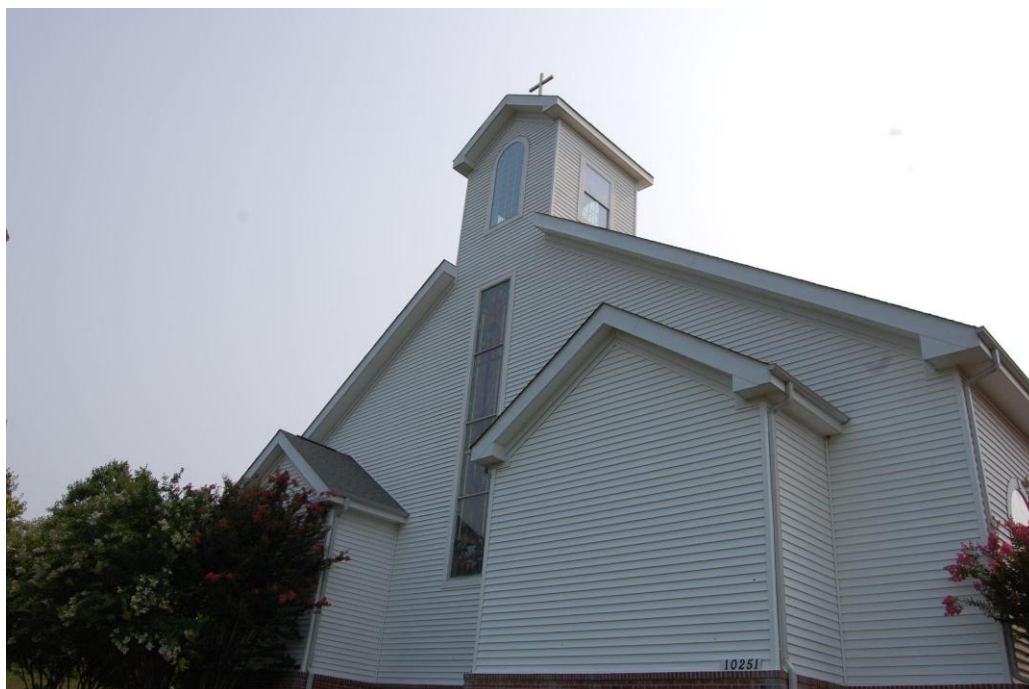
Newest portion of the Buckhall UMC, built 2007.
