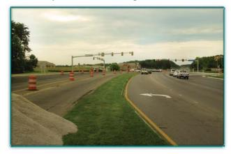
**Rollins Ford Road Improvements** - This project opened the existing four-lane section of the roadway, constructed a transition lane into the two-lane section of the roadway (between Braided Stream Drive and Estate Manor Drive) and installed a traffic signal at the Linton Hall intersection.
