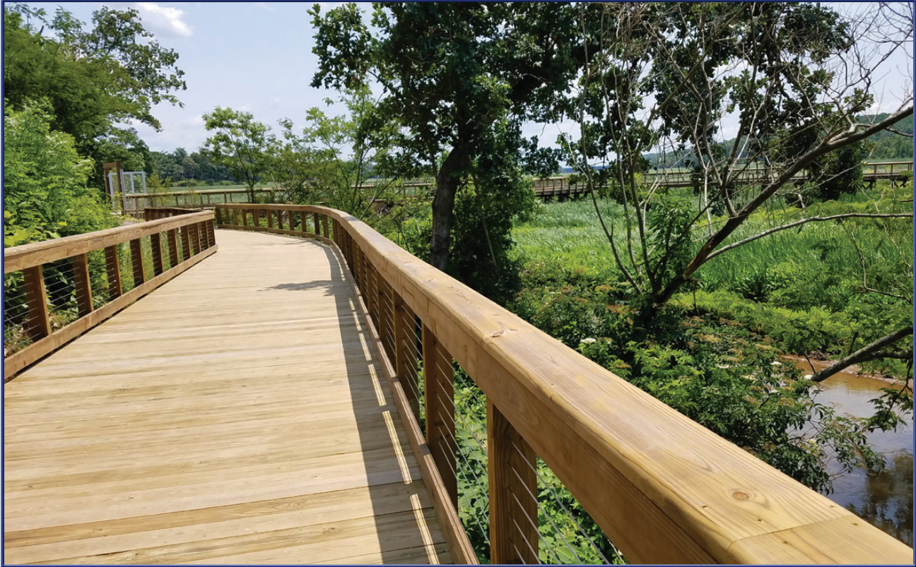
Neabsco Creek Boardwalk
