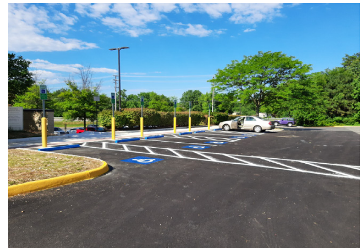
New ADA parking – Chinn Library
