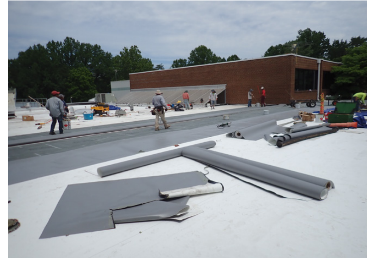
New roof – Dale City Recreation Center
