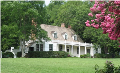
Rippon Lodge Historic Site 15520 Blackburn Road Woodbridge, VA
