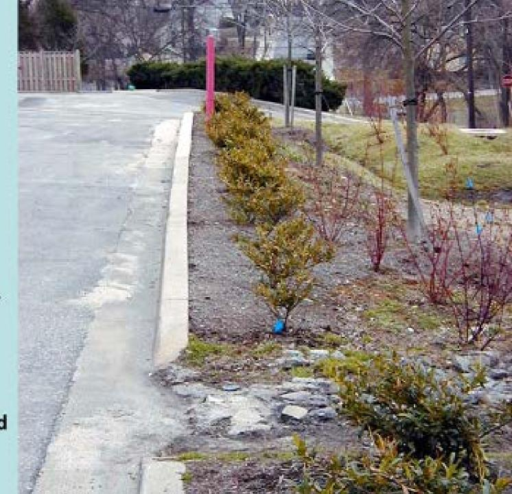
BayScaping is the utilization of deep-rooted native plants and mulch to replace turf or impermeable surfaces. This stabilizes soils and increases infiltration of stormwater.
