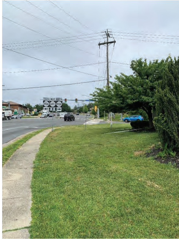
Photo east of the intersection facing west along Old Bridge Road
