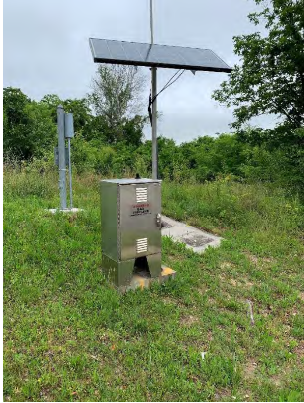
Photo of gas line northwest of the intersection
